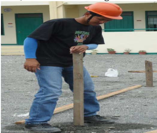
Fig.2 Putting up the stake for foundation
