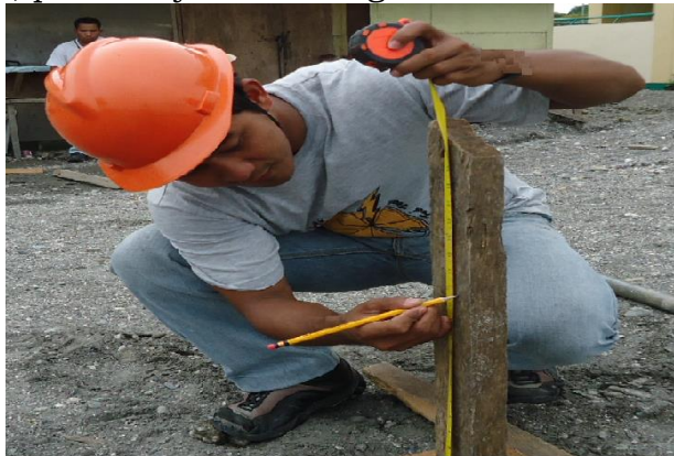
Fig.1 Determining the height of the foundation.
