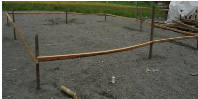
Fig. 7 A Batter board
