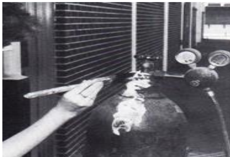
Checking gas leaks
