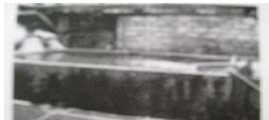
Figure 3. Concrete sand filter tanks for a small hatchery with a capacity approximately 10 m 3
