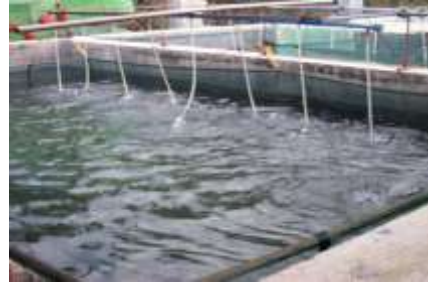
Figure 15. Tank with aerators
