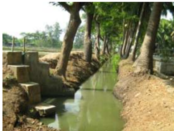
Water supply canal
